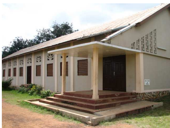
The finished church
