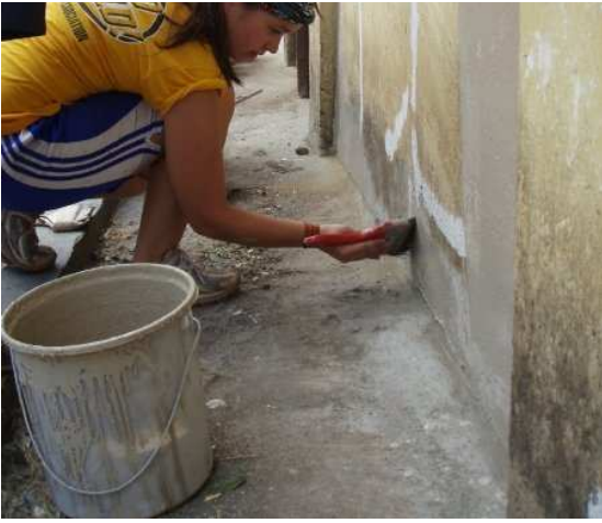
Painting the exterior
